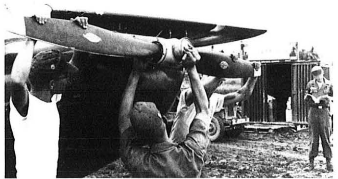
Aircraft maintenance in progress. The propeller is being replaced after a thorough inspection
